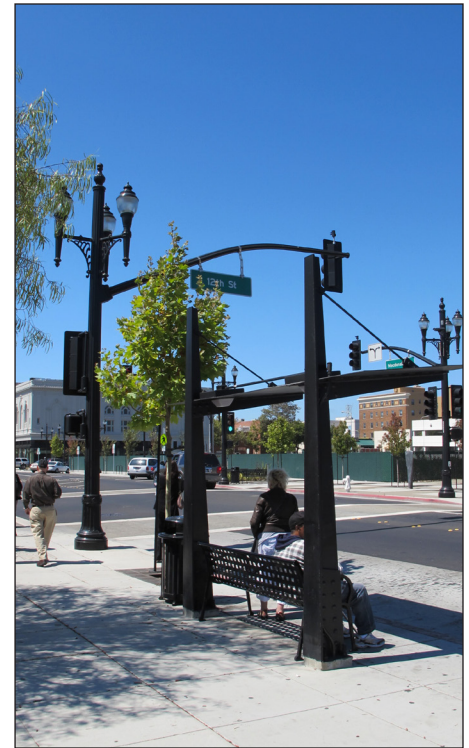
Larger poles integrated with traffic signals
